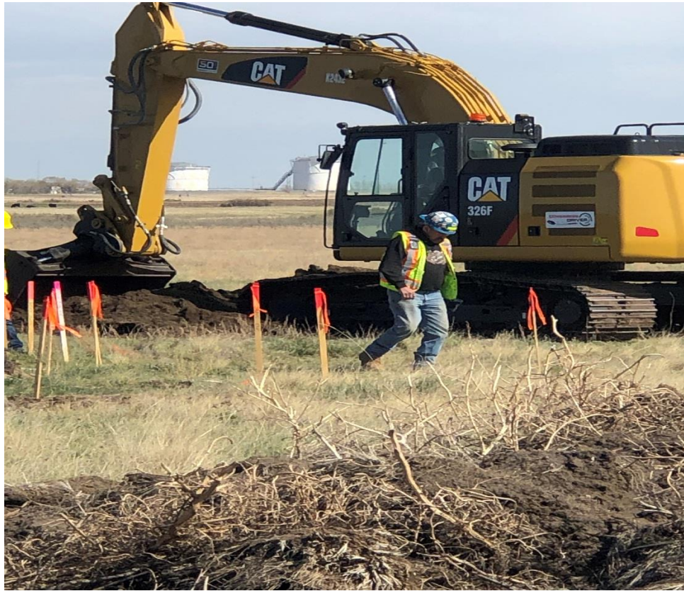
Stripping top soil from MLVB 14 to access road.
