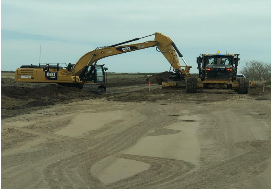
Building up access road. MKVB 14.
