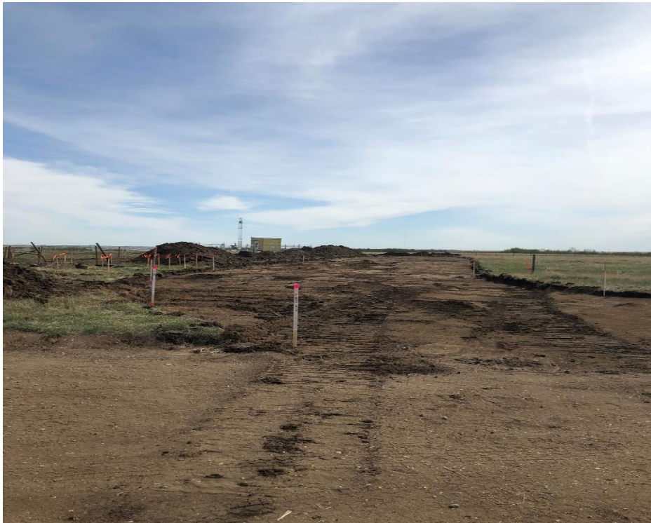
Top soil completely stripped from valve 14 to access road.
