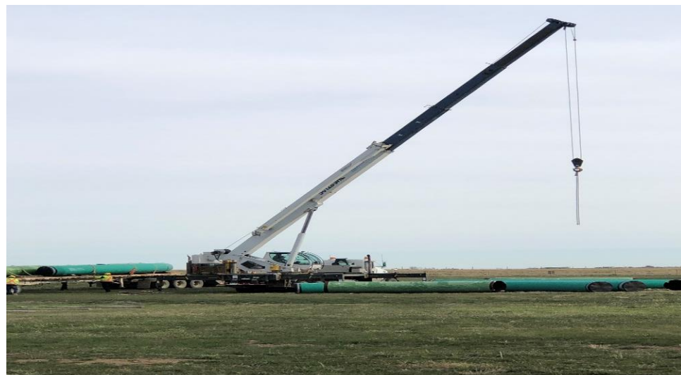
Loading pipe onto trucks with crane. Bethune pipe yard.
